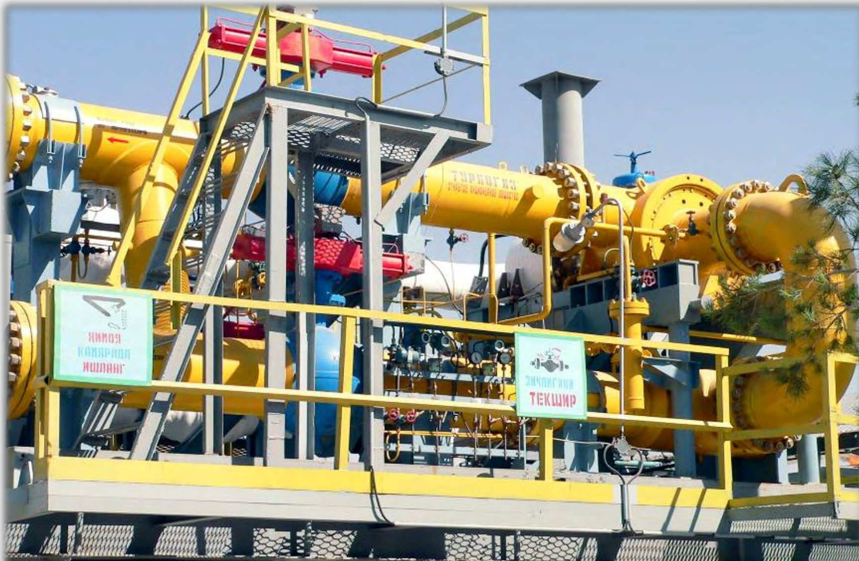
Expander –compressor unit MTDA -9,0-4,5-U1, UPBS-2 “Shurtan”,(Uzbekistan), since 2007. Active magnetic bearing.
